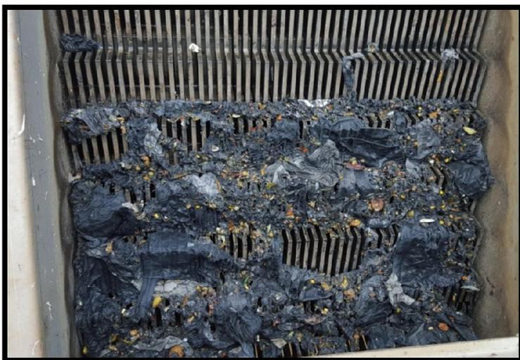
**Figure 1 Inlet step screen at Redcliffe STP**
